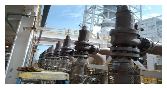
FIGURE 24: INSPECTION TO THE PSVS REPLACED POST MAY 2020 ERR CAMPAIGN LOCATED ON THE BU-DPP PLATFORM
