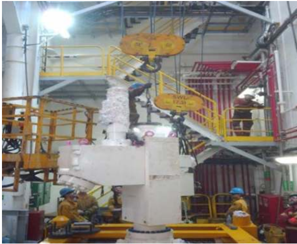
FIGURE 26: LOWERING W12 XMAS TREE FROM RIG TO WP1 FIGURE 27: OBSERVING W12 WELL TEST FLARING ON NTP RIG
