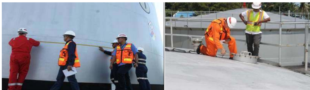
FIGURE 23: EXTERNAL TANK SHELL AND TANK ROOF INSPECTION AT PITSA FACILITY
