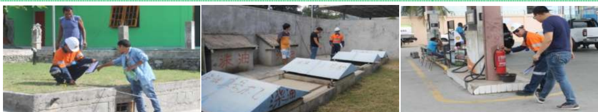
FIGURE 21: INSPECTION FROM DOWNSTREAM TEAM
